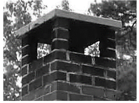
Concrete Cap Chimney Top
